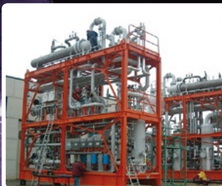
Cadiz - commissioning ed imbarco impianti off-shore Cadiz - Commissioning and boarding offshore installations
