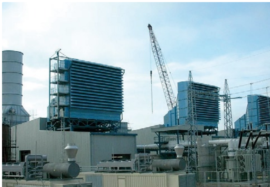
Nigeria supervision al montaggio di air-intake donaldson Nigeria - Assembly supervision air-intake Donaldson
